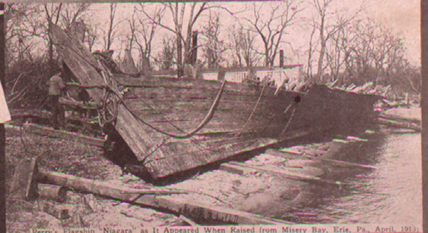
Perry's Flagship "Niagara" as It Appeared When Raised from Misery Bay, Erie, Pa., April, 1913.
