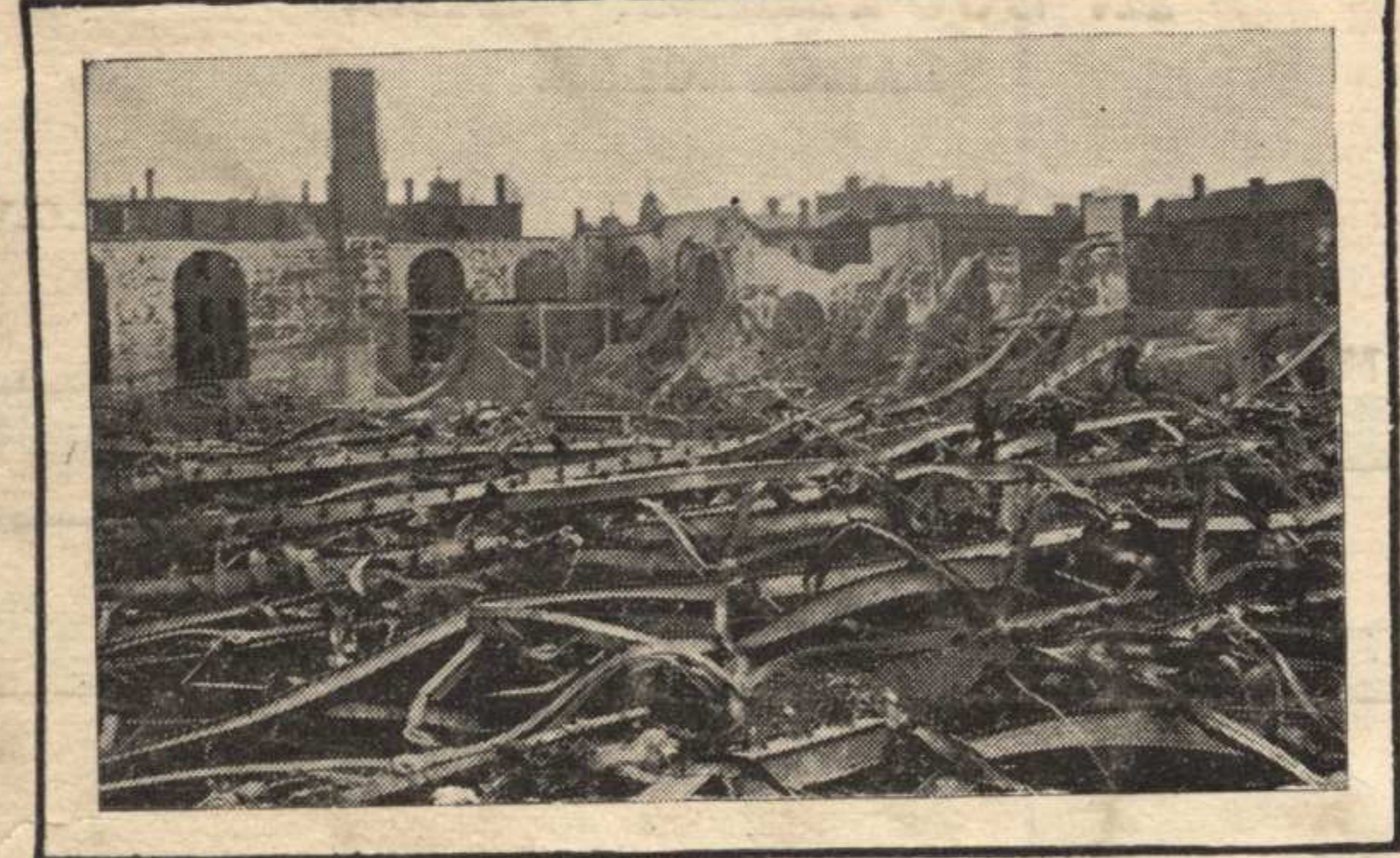
DESTROYED BY FIRE APRIL 4 TH 1900.
